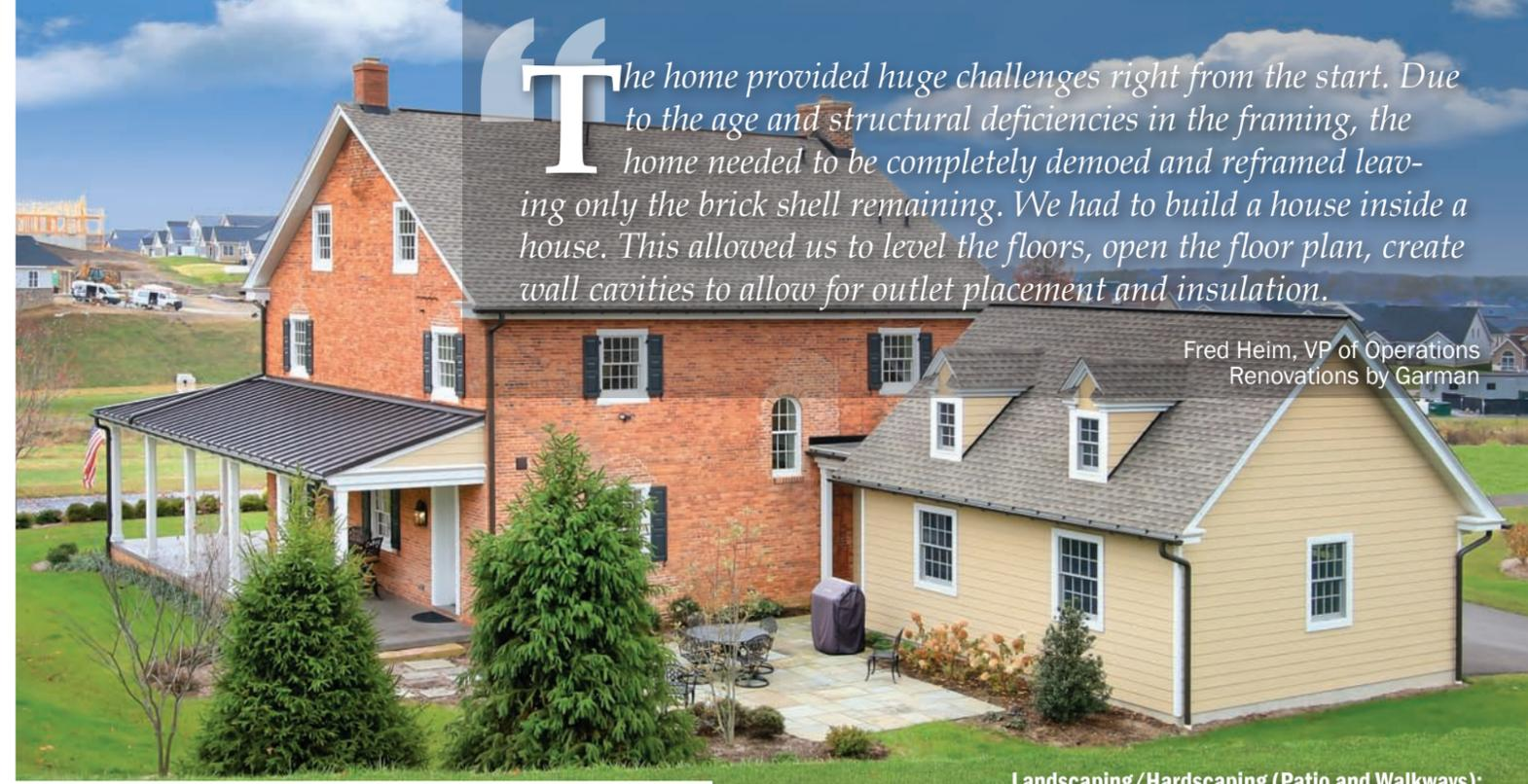
The home provided huge challenges right from the start. Due to the age and structural deficiencies in the framing, the home needed to be completely demoed and reframed leaving only the brick shell remaining. We had to build a house inside a house. This allowed us to level the floors, open the floor plan, create wall cavities to allow for outlet placement and insulation.
